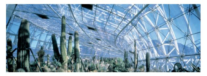
sgg DIAMANT is a unique colourless ("extra-white") float glass with a very low iron oxide content. As a result the glass has a very high light transmittance level and is significantly less green in appearance when compared to ordinary float glass. It is therefore the only clear glass which allows a natural and true reproduction of white and pastel colours when enamelled, lacquered or screen printed.
